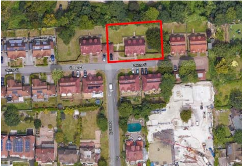
Figure 2: Aerial street view within the surrounding streetscene
